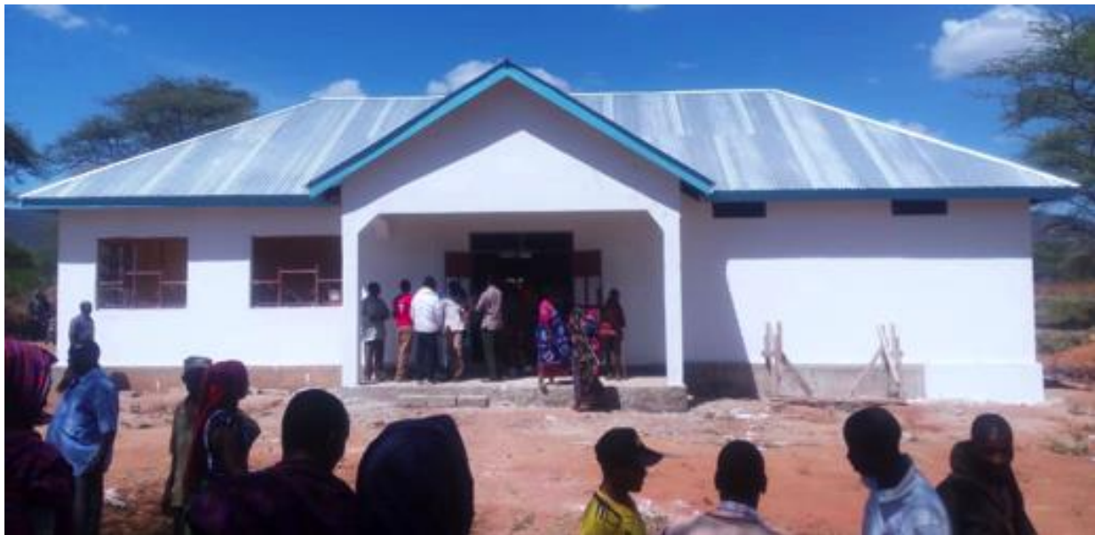
New police station in Yaeda Chini Village built with a combination of district government funding and contribution of revenue from Hadza communities. Photo Credit: Carbon Tanzania
