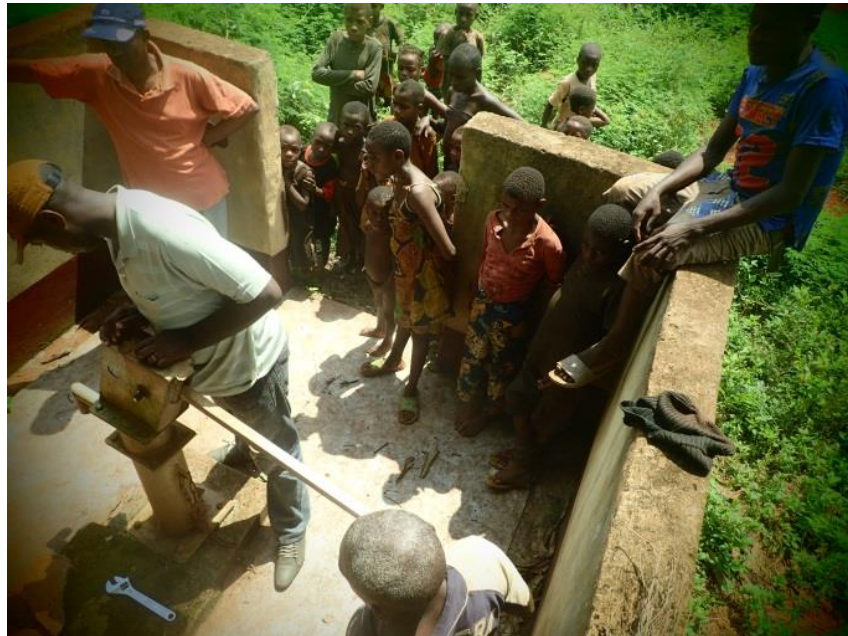
Feasibility work on well rehabilitation in Lobéké, Cameroon. Credit: WWF
