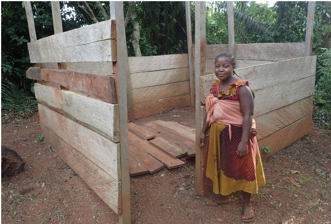
Household latrine constructed by community members with technical support from WWF health scouts, in Lobéké, Cameroon. Credit: Olivier Njounan, WWF
