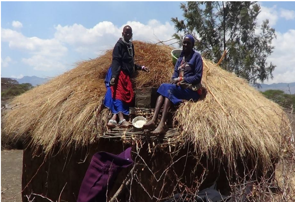
Maasai women on top for the roof installing the chimney
