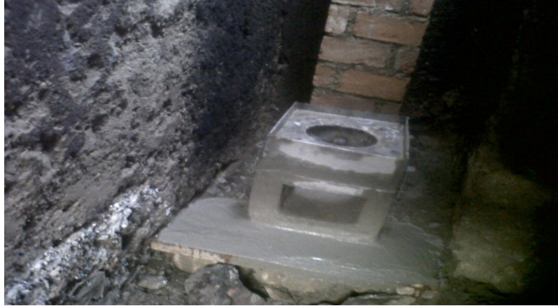
A cookstove installed in a house
