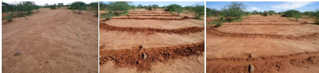
Gully healing and reseeded work, meibae
