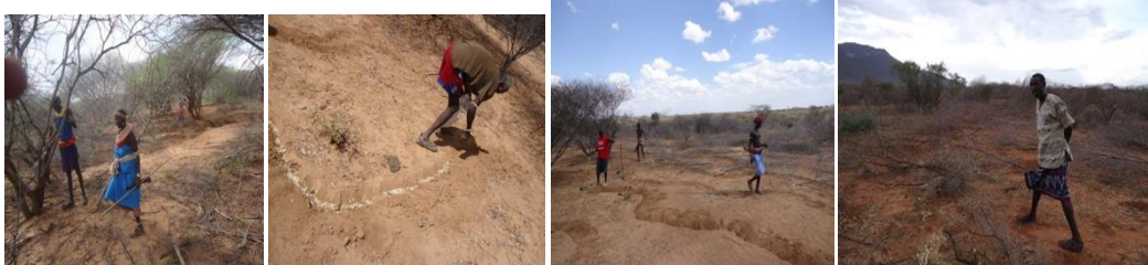
Clearing and reseeding work above
