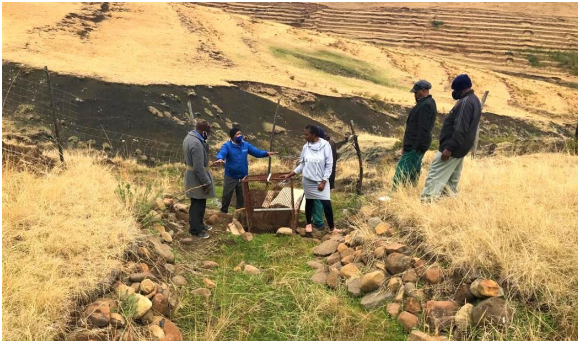
Msukeni Spring Site Inspection, South Africa, September, 2020. Photo credit: Zola Mbuyana, ANDM
