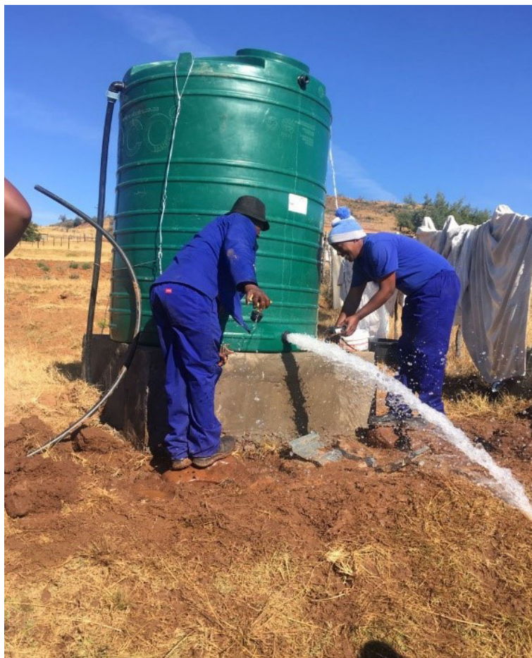
Water monitors connecting pipes from the tap to the tank for community members to collect. Photo credit: Mzingisi Nyhodo, CSA
