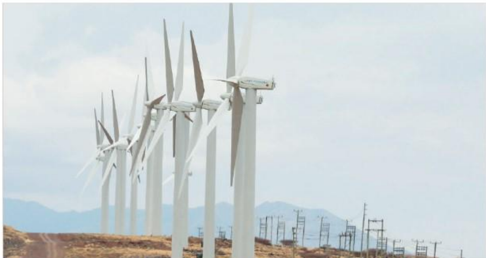
Wind turbines at the Lake Turkana Wind Power project (LTWP) in Loiyangalani, Marsabit county, Northern Kenya/FILE
